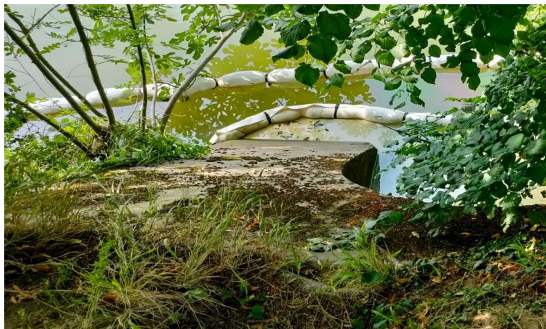
Barrage flottant (photo inspection)
