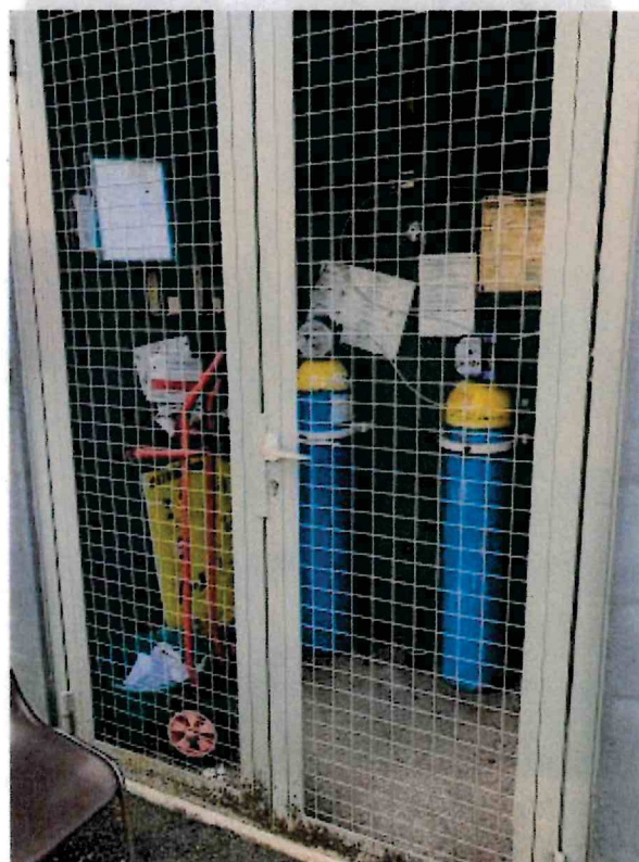
STOCKAGE CHLORE GAZEUX
