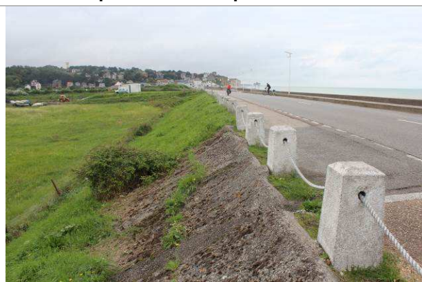
Parement aval digue route
