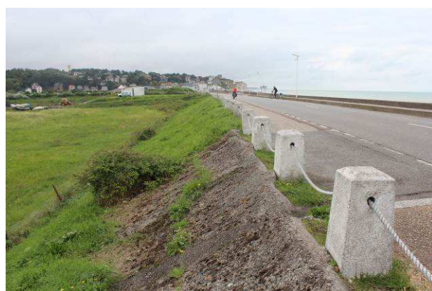
Parement aval digue route
