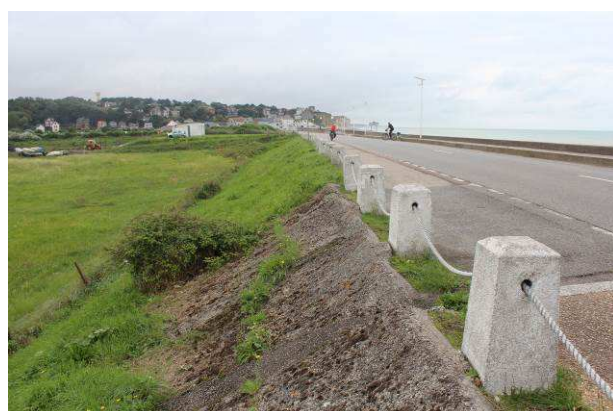
Parement aval digue route
